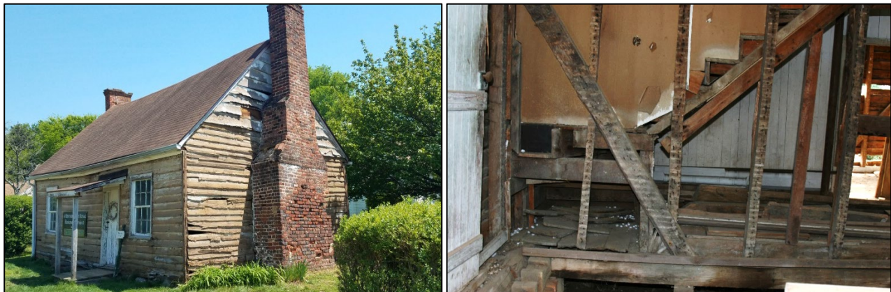
Restoration project in progress, the Murray House, circa 1750.
